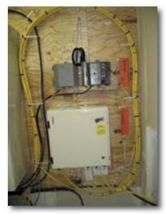
At the Building Communication Gateway. Note the gentle bending radius of the fiber ducts.
